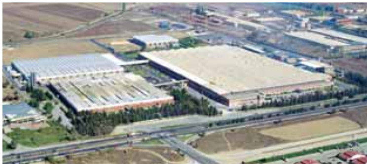
Refrigerator Plant Eskişehir
