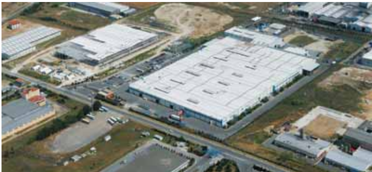
Tumble Dryer and Electric Motors Plant. Çerkezköy, Tekirdağ
