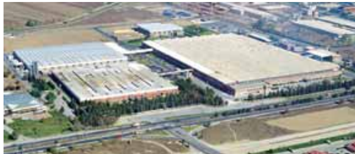
Refrigerator and Compressor Plant Eskişehir
