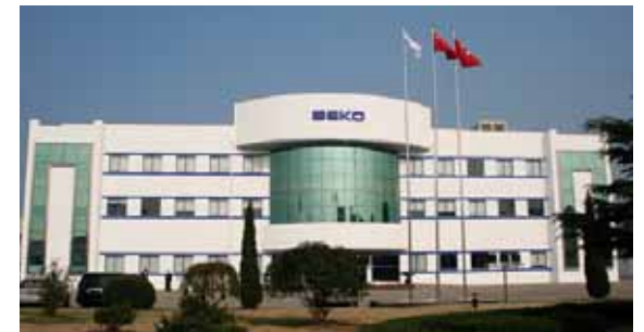
Beko Electrical Appliances Washing Machine Plant China
