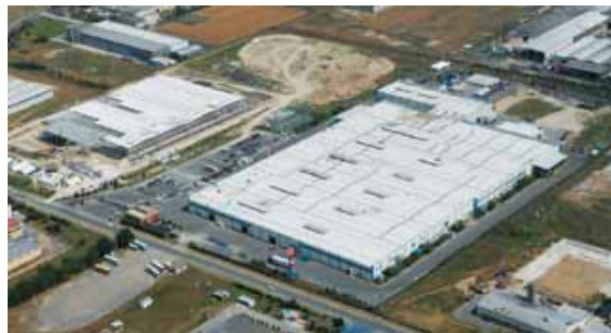
Tumble Dryer and Electric Motors Plant Çerkezköy, Tekirdağ
